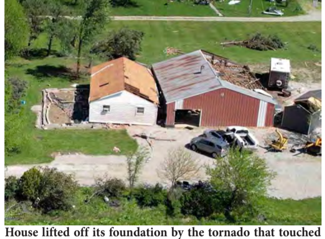
House lifted off its foundation by the tornado that touched down south of SR 613 on Rd. 151 near Melrose. Drone photo by Engaging Exposures Photography.
