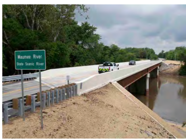
Local residents and brothers, John and Tim Walk, were the first to cross the newly constructed US 127 bridge following a ribbon cutting on Friday, May 17, 2024
