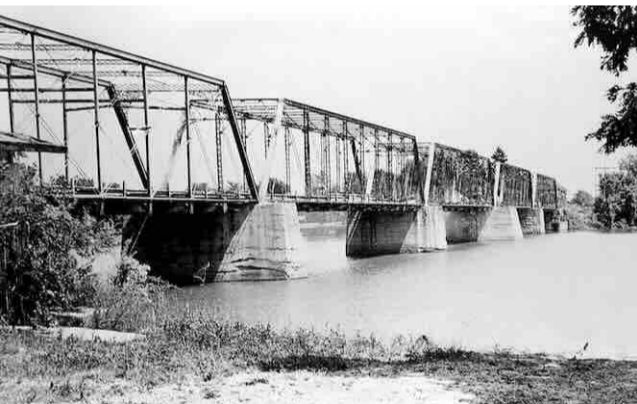
The old Five Span Bridge east of Junction as it appeared in 1957. The bridge opened in 1875 and was demolished in summer 1983. The new bridge was completed in December 1984.
